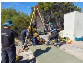
Preparing to descend into the 5.25m Engine Bay
