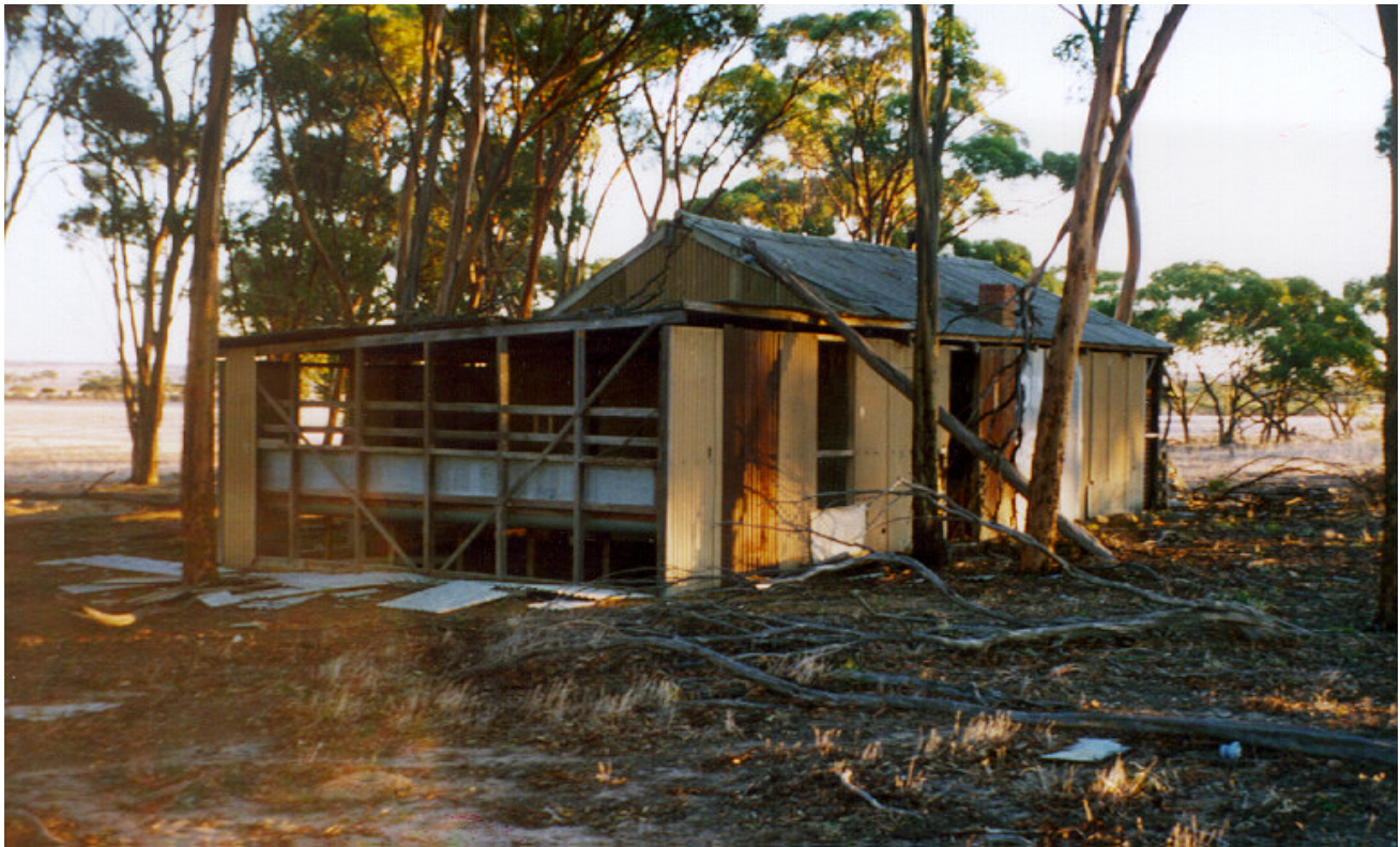
Ablution and laundry building, Ardath Ammunition Depot, Shire of Bruce Rock Photo: B Bridges / H Birch
